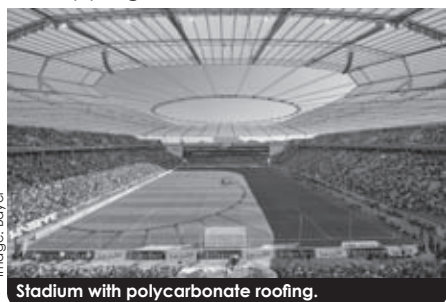
Stadium with polycarbonate roofing.
